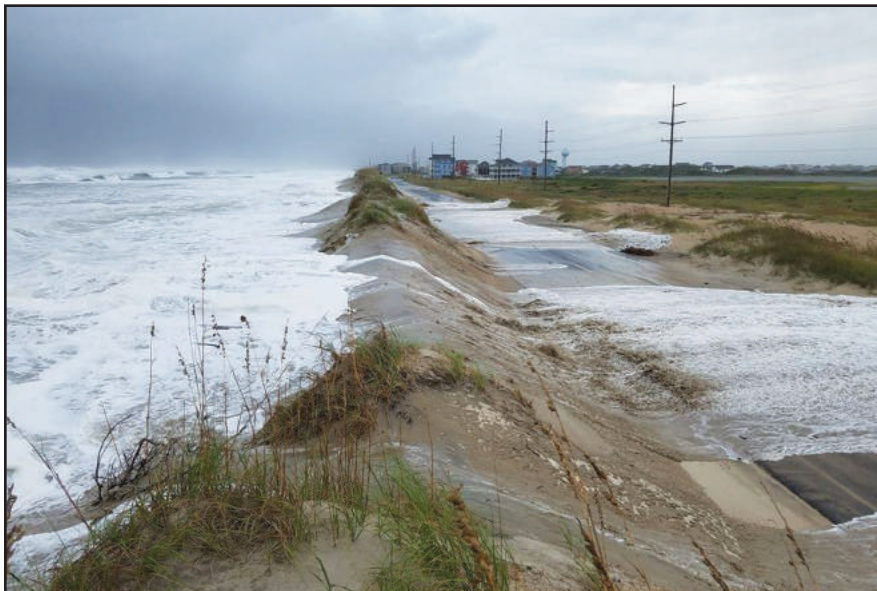
Wash over at Sandy Bay on HWY 12 close to the Hurricane Isabel breach of 2003 (Reprint from NC DOT NC 12 Facebook)
